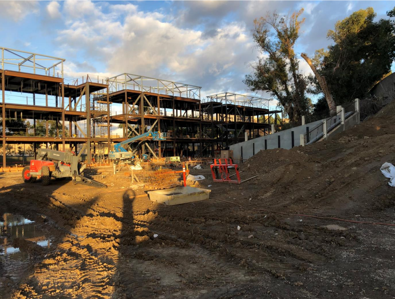
Restorative Care Village
