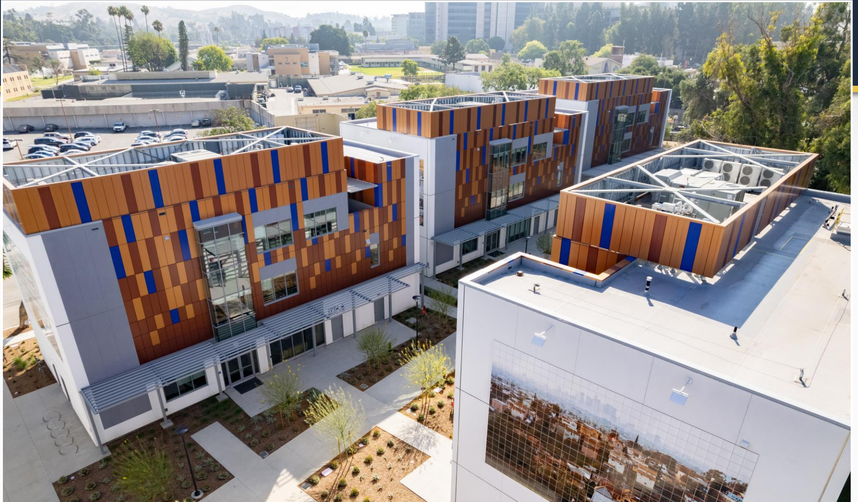
Restorative Care Village Projects
